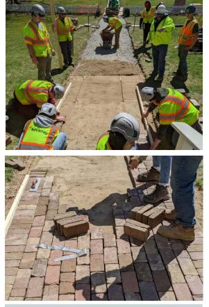
After tamping down the gravel substrate and a layer of dirt, students begin relaying brick using guides to keep the bricks evenly spaced and straight.
