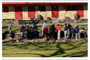
TSCT students work on removing and restacking stones during the reconstruction of the stone wall in front of the Rock Ford Barn.
